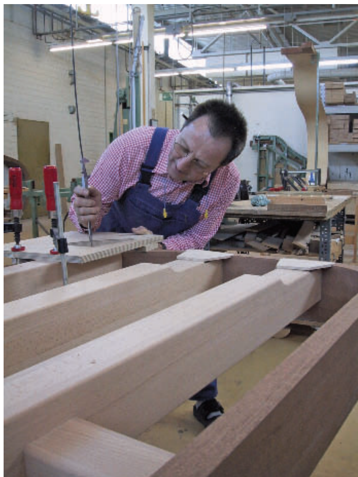
Photo 6 — Sauter craftsman in Germany, installing the 275 beams with dovetail joints.
